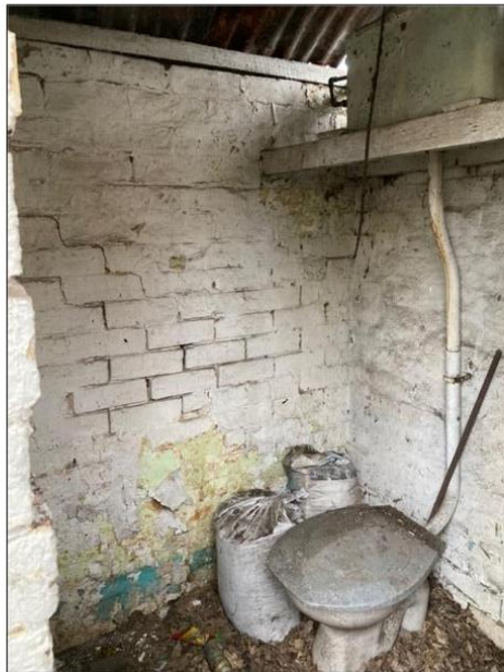
Figure 9: The fit-out to the outhouse.
