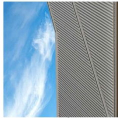
metal roof, light colour, colorbond/corrugated iron
