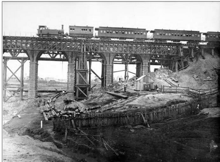
Figure 2: Long Cove Creek Viaduct Whipple Truss under construction (c. 1886). State Archives NSW
