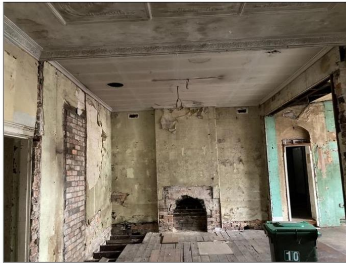
Figure 20: The main shop area, looking east towards the brick hearth. Note the difference in the ceilings, indicating it was likely originally two rooms.
