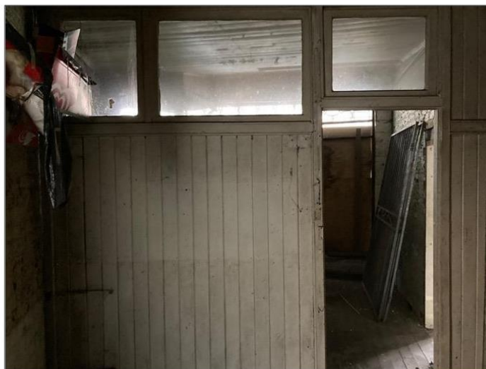
Figure 25: Looking towards the front of the small shop area.
