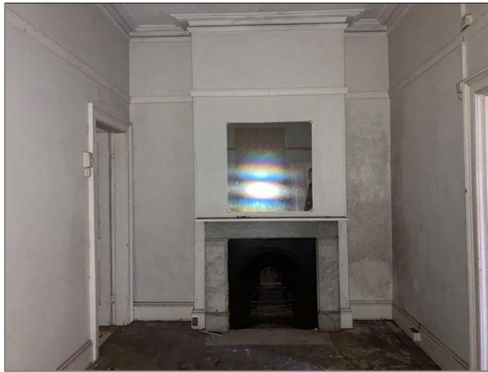
Figure 31: Living room, looking towards the only intact fireplace in the building.
