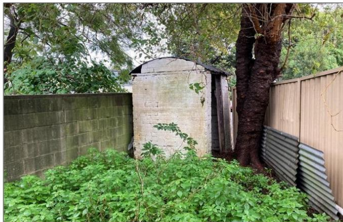
Figure 8: The brick outhouse and vegetation patterns to the rear yard.
