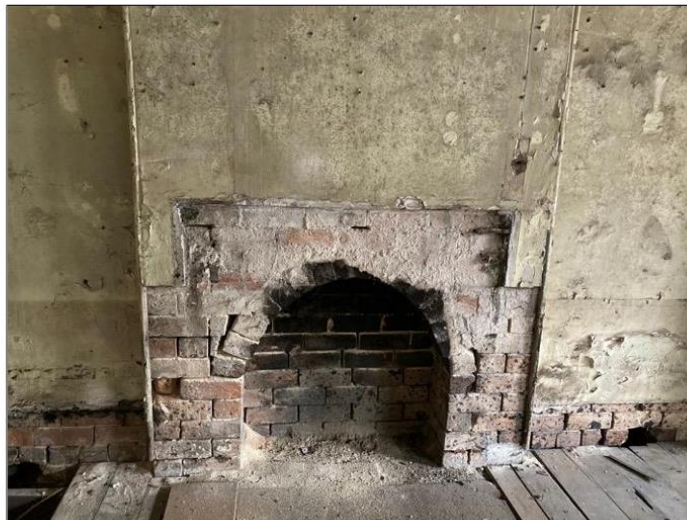
Figure 21: Close-up view of the remnant brick hearth with the mantelpiece and insert removed.
