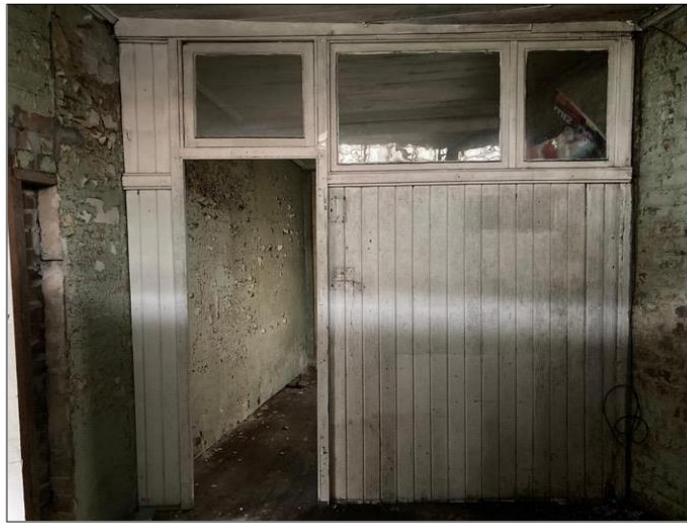
Figure 24: The second, smaller shop showing internal dividing wall.
