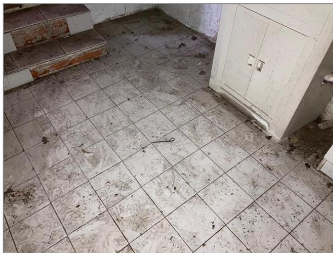
Figure 36: The tiled floor finish to the bathroom/laundry.
