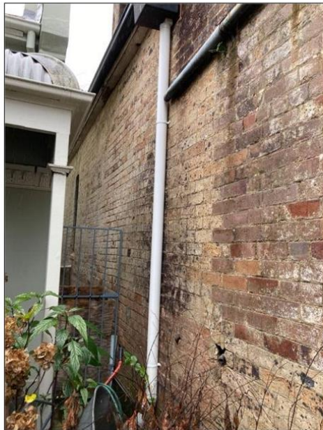
Figure 16: Unpainted brick wall to the western elevation of the principal building.
