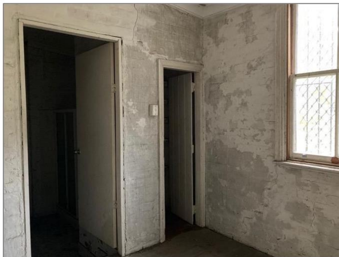
Figure 32: Kitchen, looking towards pantry and the bathroom/laundry.
