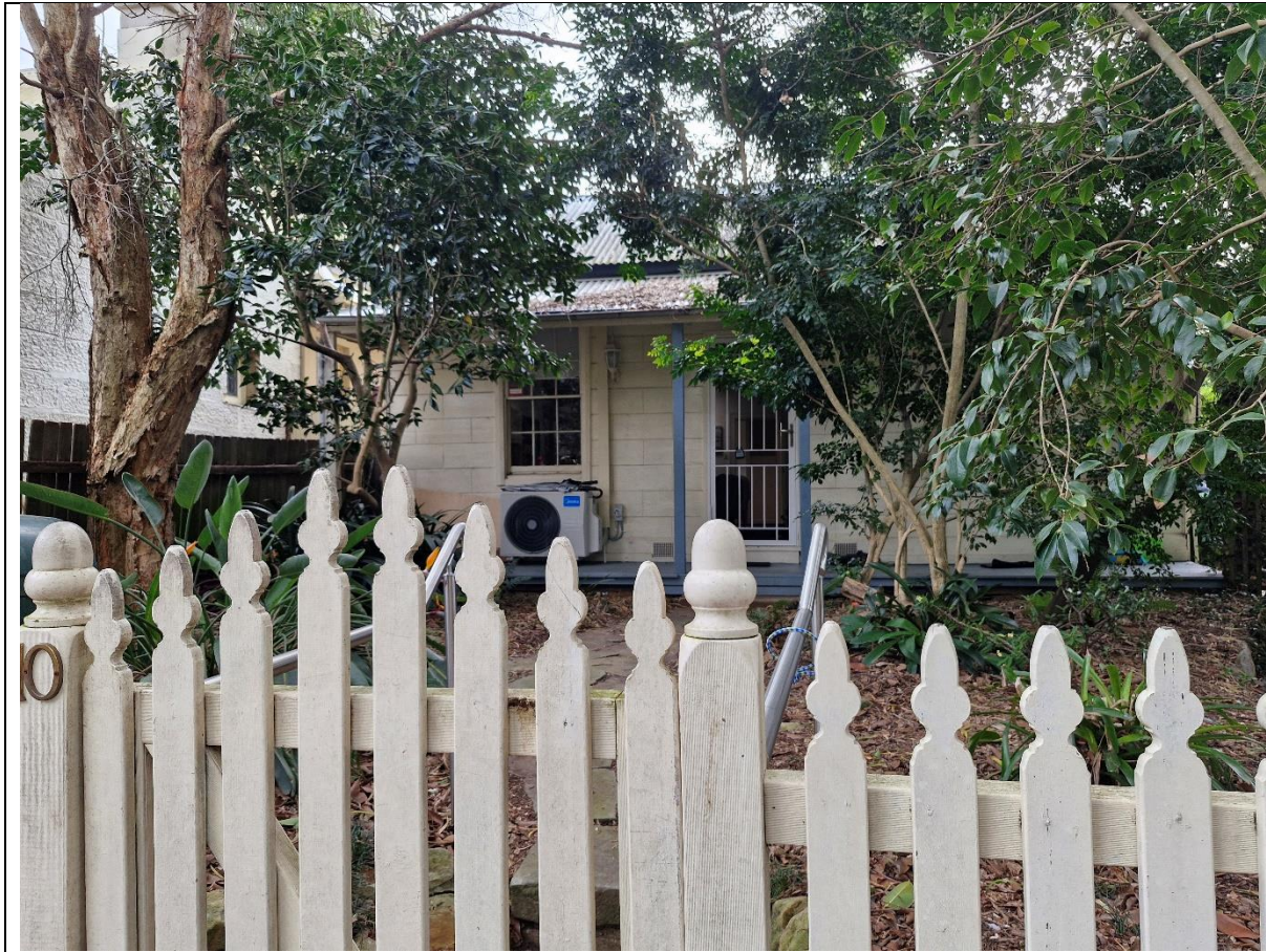
Figure 2: Photo of subject site as viewed from Waterview Street
