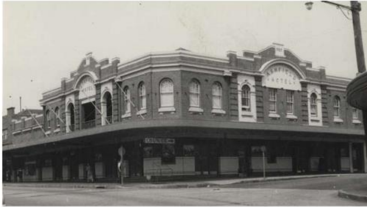
Figure 2.15 The Ashfield Hotel in 1960
