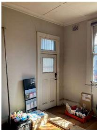
Figure 10.14 Current northern store with door to the balcony. This room will remain as is
