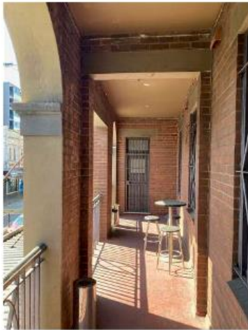
Figure 7.10 First floor balcony – end doors will be retained along with the central window
