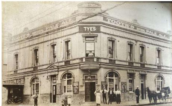
Figure 2.4 The first Ashfield Hotel, undated
