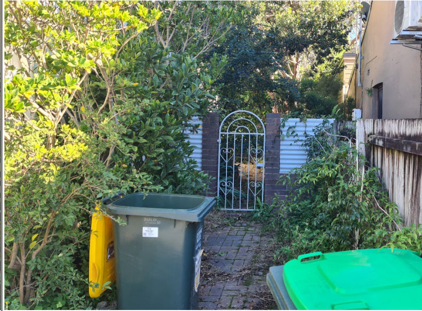
PHOTOGRAPH 14: RESIDENTIAL TERRACE (71 CROWN ST)
