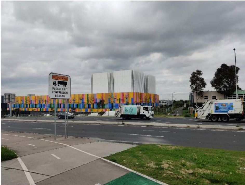
View from Campbell Street – opposite side of the site
