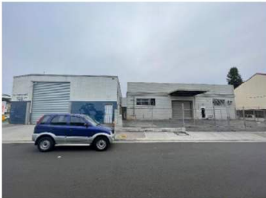
View from Crown Street of 85 Crown Street (left) and 116 Princes Highway (right)
