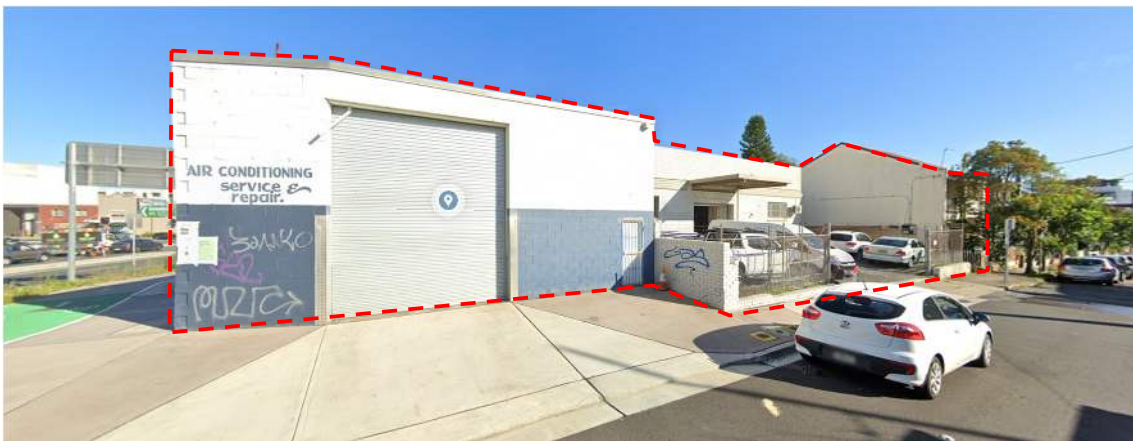
Figure 6: Site viewed from Crown Street
