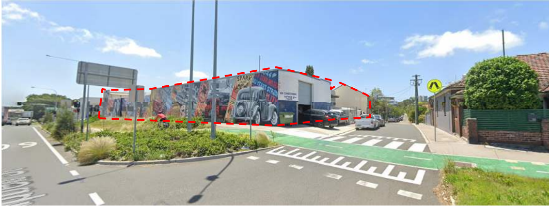
Figure 5: Site viewed from Campbell Street and Crown Street
