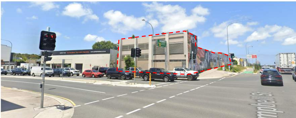
Figure 4: Site viewed from Campbell Street and Princes Highway
