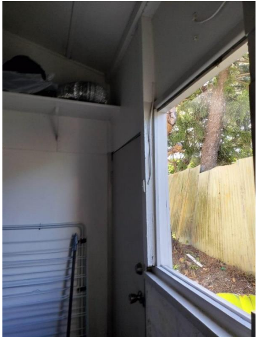
Figure 4-21: Annex at rear of 77 Crown Street. Source: Curio 2023
