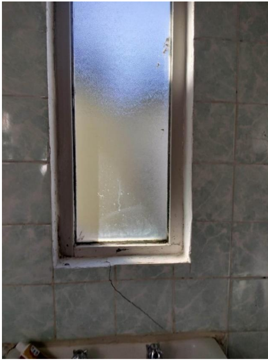
Figure 4-29: Bathroom in annex of 75 Crown Street. Source: Curio 2023
