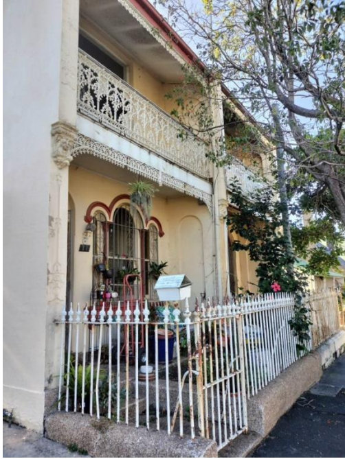
Figure 4-7: Front façade of 77 Crown Street, facing northwest. Source: Curio 2023
