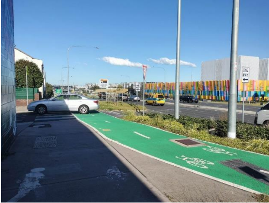
Figure 4-2: Taken from the study area, facing southeast down Campbell Street. Source: Curio 2023
