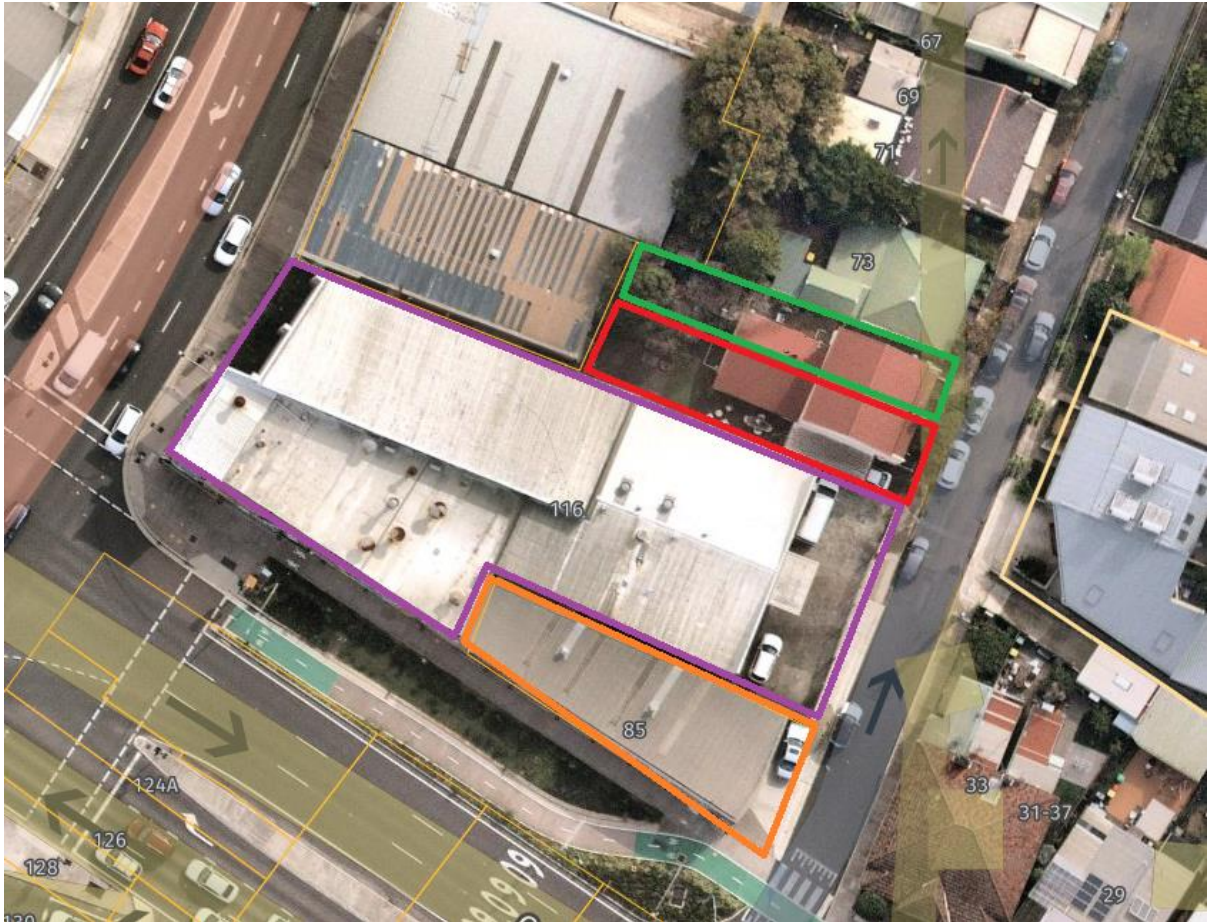
Figure 4-1: The buildings comprising the study area. 75 Crown Street in green, 77 Crown Street in red, 116 Crown Street in purple and 85 Crown Street in orange. Source: NearMap 2023 with Curio markup
