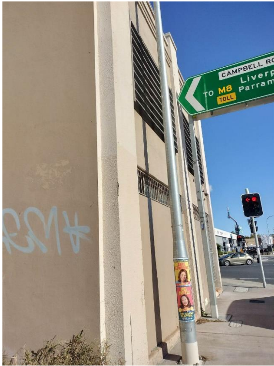
Figure 4-47: Rear of warehouse on Princes Highway frontage, facing south. Source: Curio 2023
