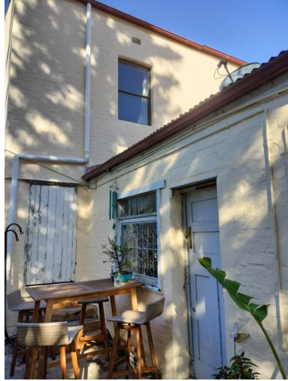
Figure 4-42: Annex at rear of 75 Crown Street, with door leading to backsteps at the left. Source: Curio 2023
