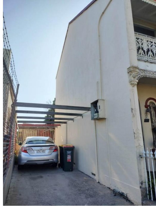
Figure 4-24: Southern wall of 77 Crown Street with carport. Source: Curio 2023
