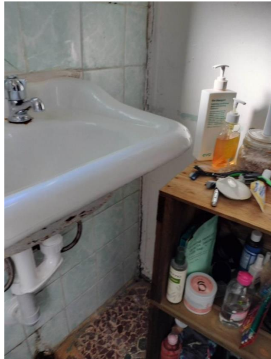
Figure 4-30: Bathroom in annex of 75 Crown Street. Source: Curio 2023
