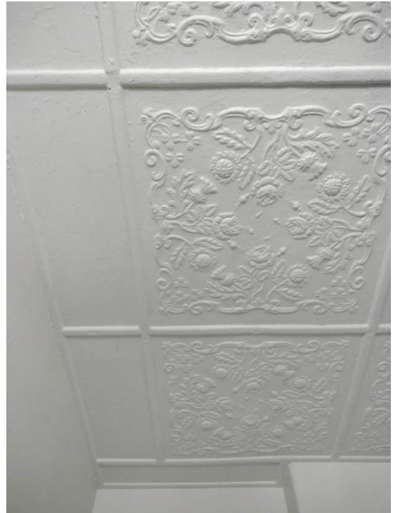
Figure 4-28: Plaster ceiling of ground floor of 75 Crown Street. Source: Curio 2023
