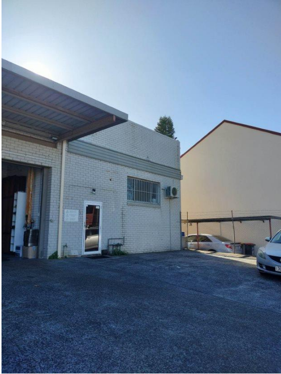
Figure 4-43: Brick warehouse on Crown Street frontage, with terraces in background, facing northwest. Source: Curio 2023
