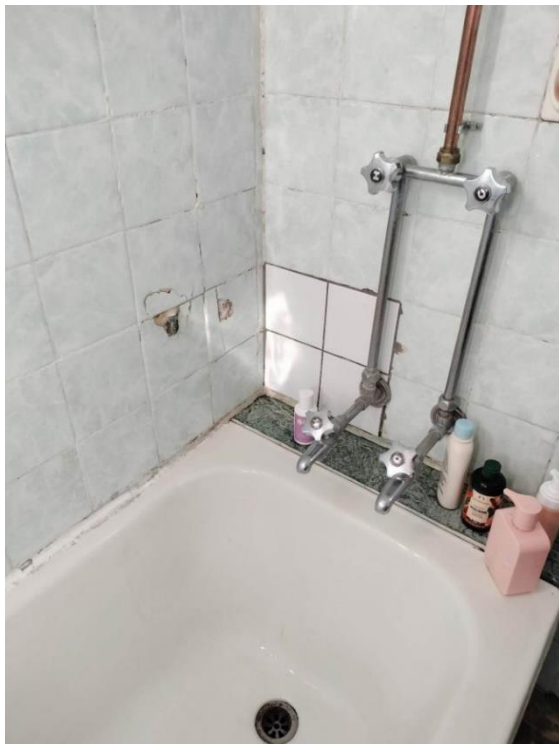
Figure 4-31: Bathroom in annex of 75 Crown Street. Source: Curio 2023
