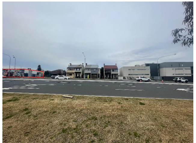
Development east of the site on Campbell Street (site in red)
