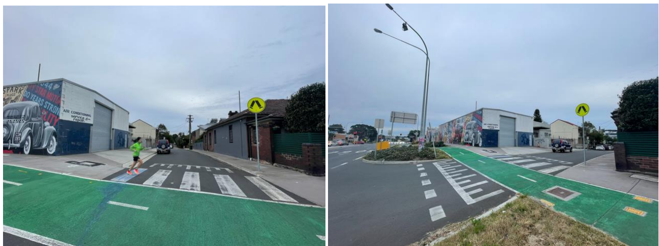
Figure 4 – Off-Road Cycle Paths on Campbell Street
