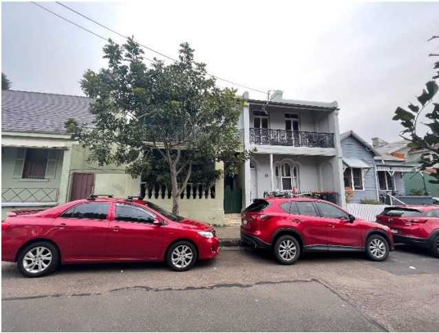
Terraces viewed from Crown St
