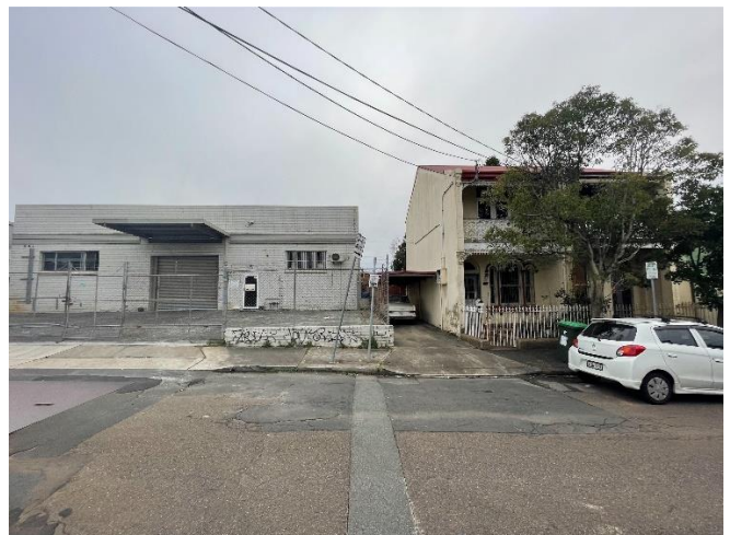
View from Crown Street of 116 Princes Highway (left) and 75 Crown Street (right)
