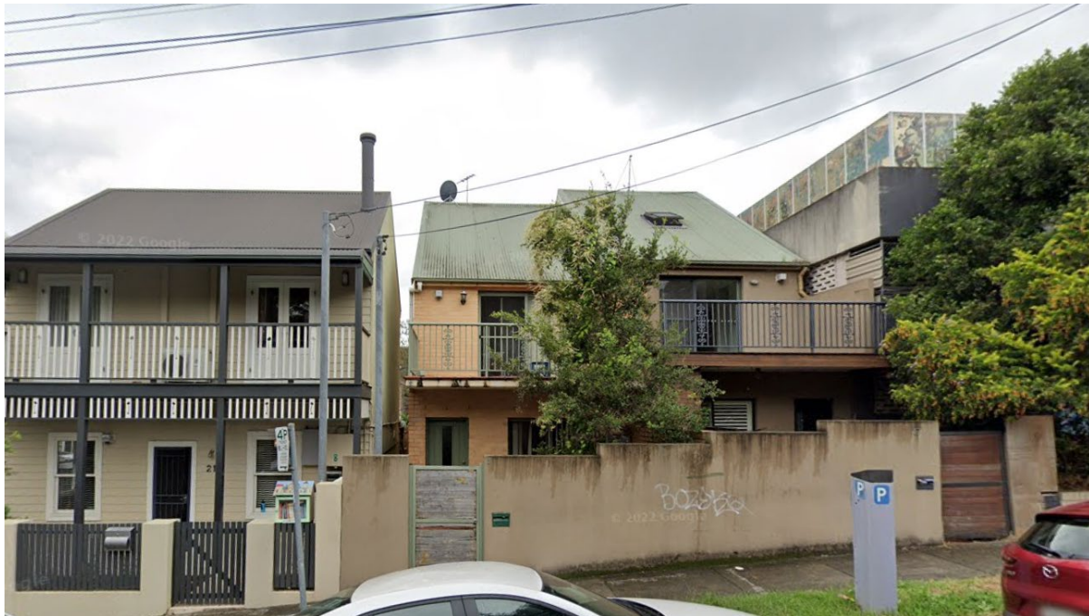
Figure 3: View of proposed site from Waterloo Street
