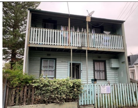
Figure 5: Existing front view of subject site
