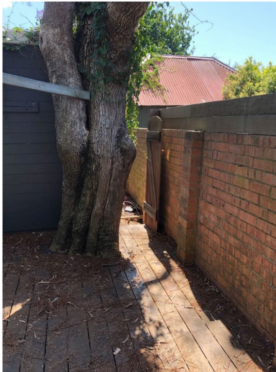
Plate 1: Image showing Tree 1 in relation to the brick wall that will be moved closer to Tree 1. P. Vezgoff.
