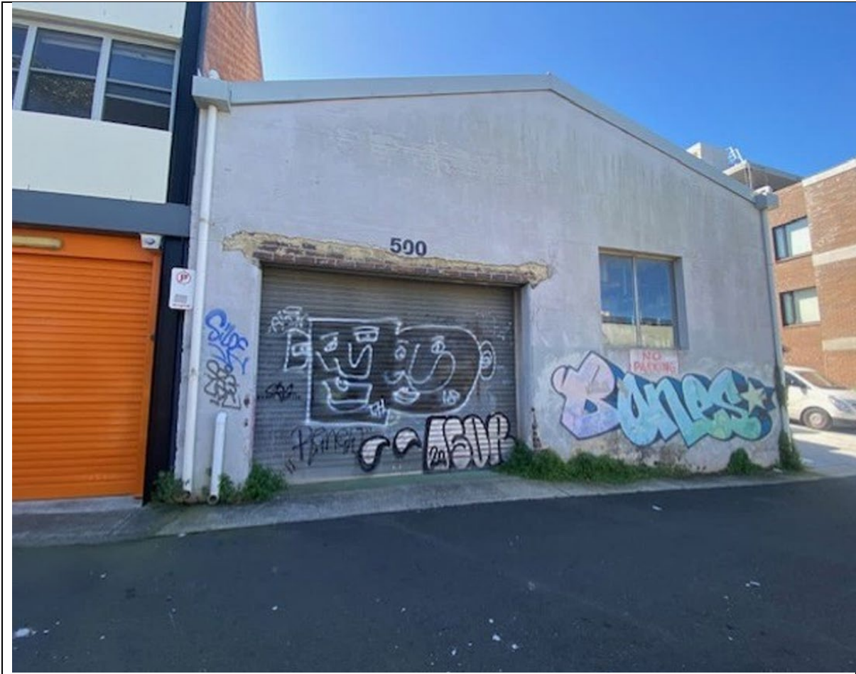
Figure 2 – Site Photo (Durham Lane Street Frontage)
