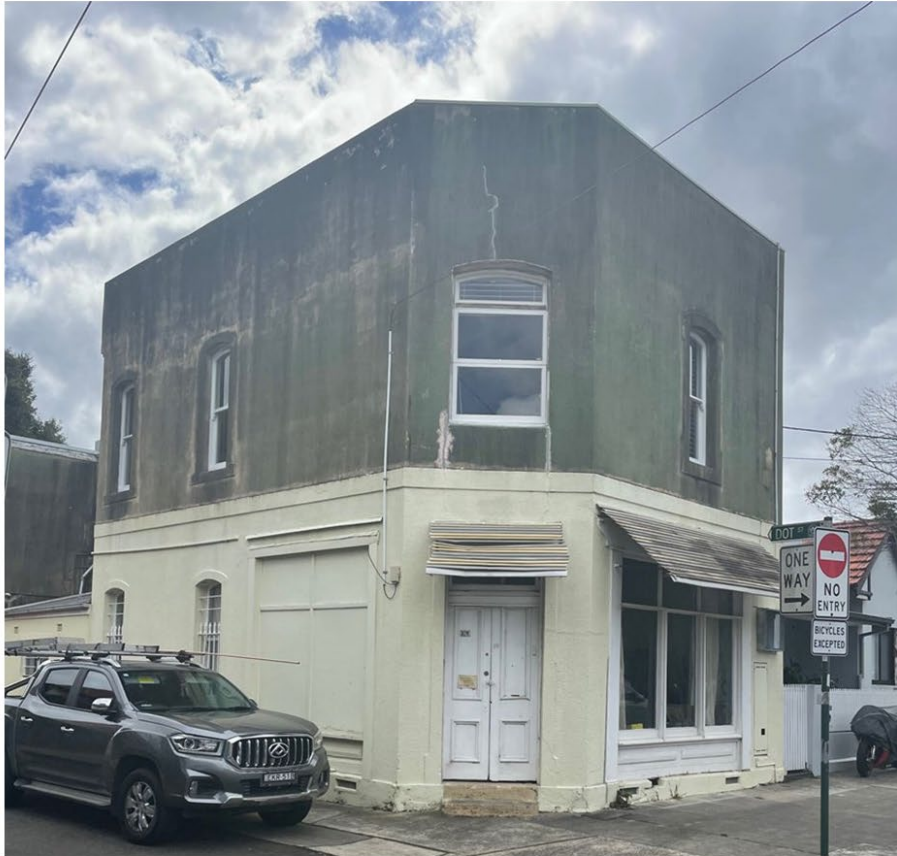
Figure 2: 19 Roberts Street Marrickville, site visit 22/09/2023
