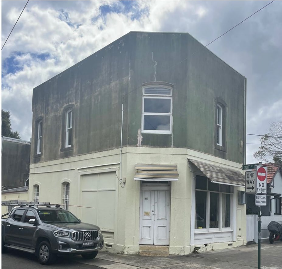
Figure 2: 19 Roberts Street Marrickville, site visit 22/09/2023
