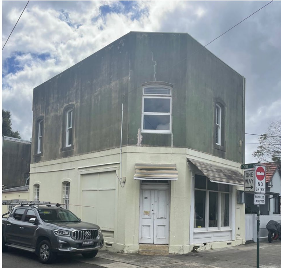
Figure 2: 19 Roberts Street Marrickville, site visit 22/09/2023
