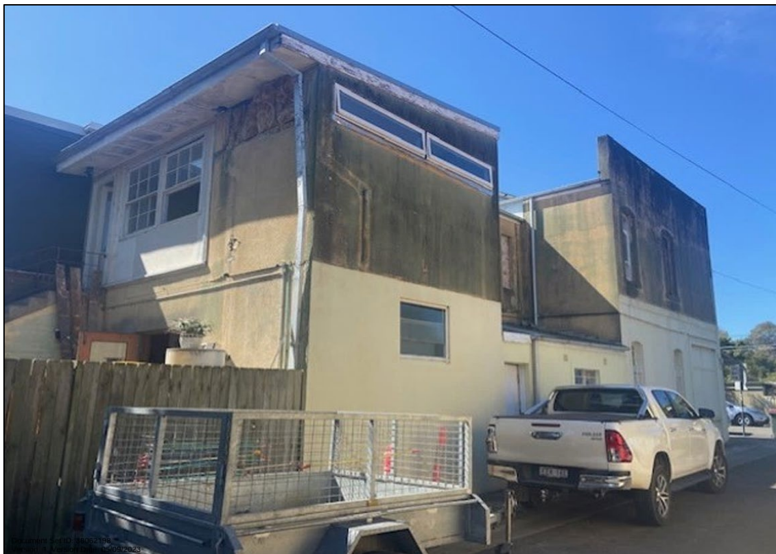
Figure 1 – Site Photo (Dot Street Frontage)
