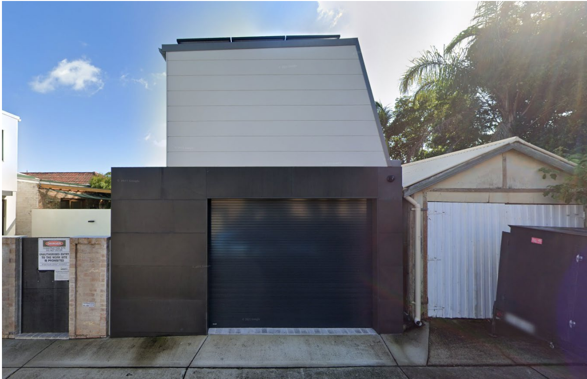
Figure 4 - No. 22 South Street's two-storey outbuilding as visible from Dot Street and adjoining the subject site
