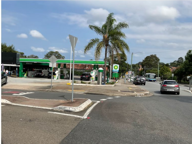
Figure 7: The BP Service Station (at left) looking east along Ramsay Street
