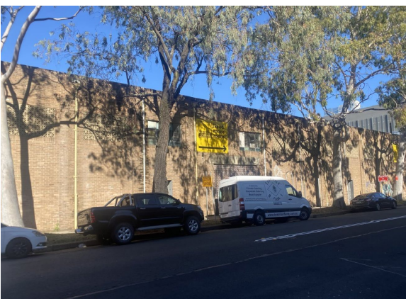
Picture 5 View of the 11A Edinburgh Road site from Smidmore Street
