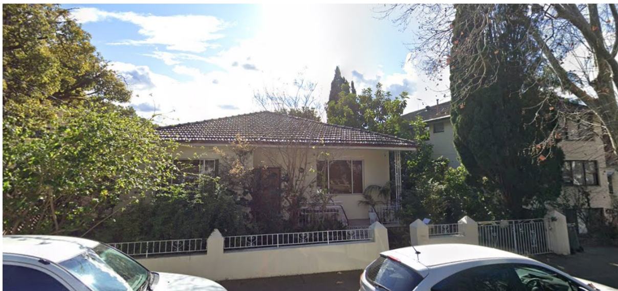
Figure 2: The Subject Site at 77 Glassop Street
