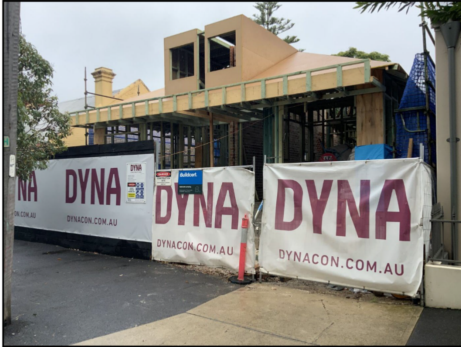
Figure 8: Subject site with DA/2022/0365 under construction
