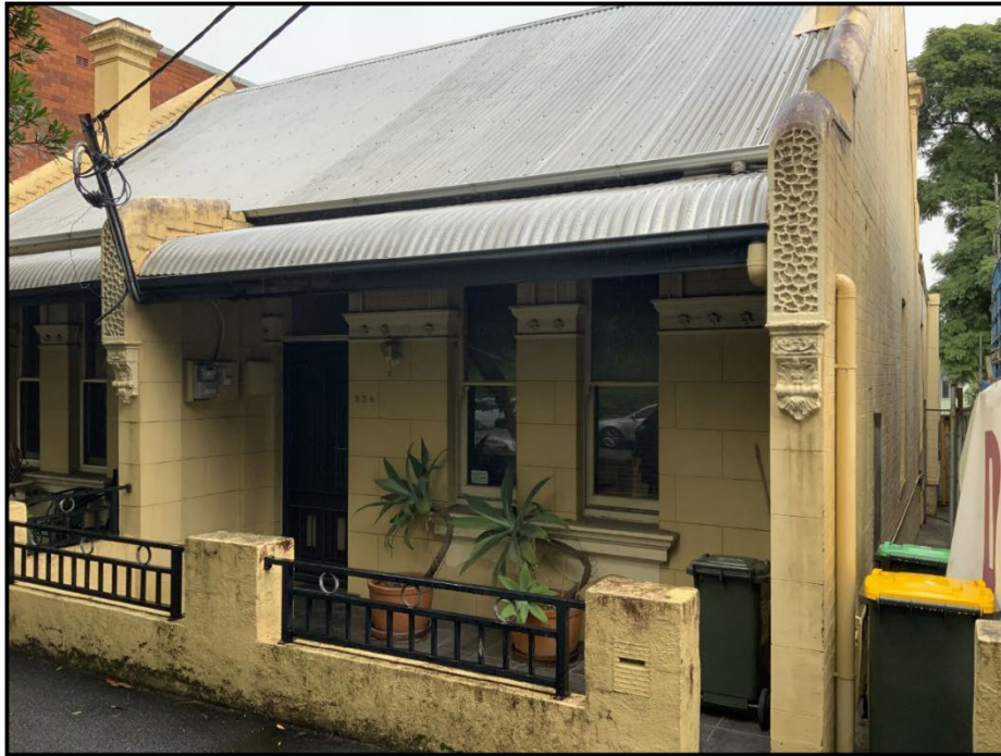
Figure 5: 222 and 224 Norton Street, semis to the south of the subject site with a similar frontages and lot sizes as the proposed lot frontages/sizes
