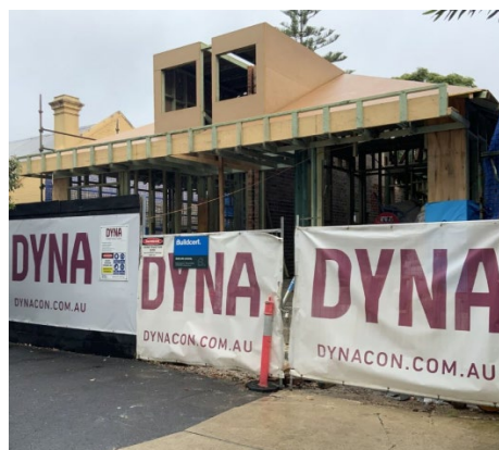
Figure 2 - Photo of subject site
