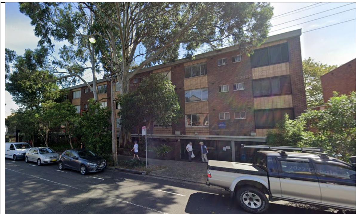
FIGURE 4: VIEW OF EXISTING BOARDING HOUSE AT 121-125 BOOTH STREET ANNANDALE
