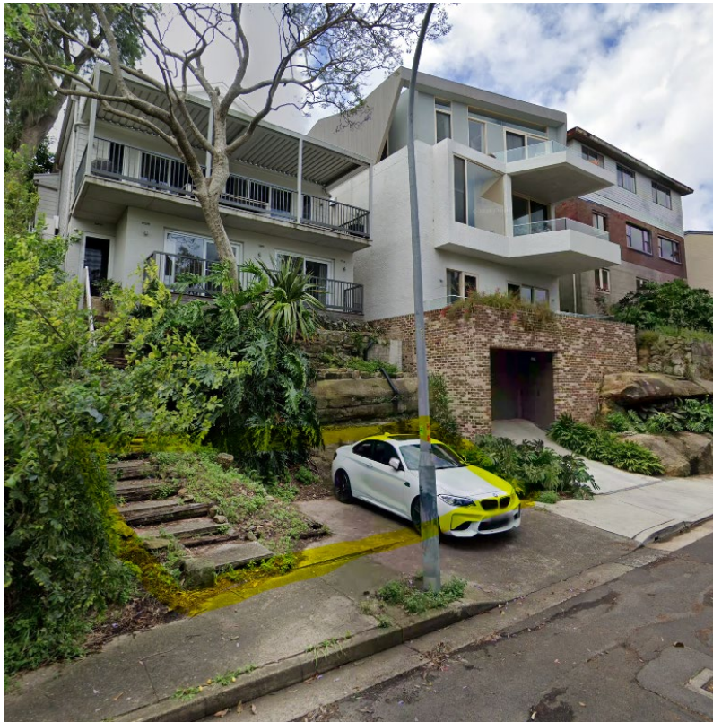
Photograph 1 - Depiction the subject lot (highlighted) and the eastern section of Yeend Street.
