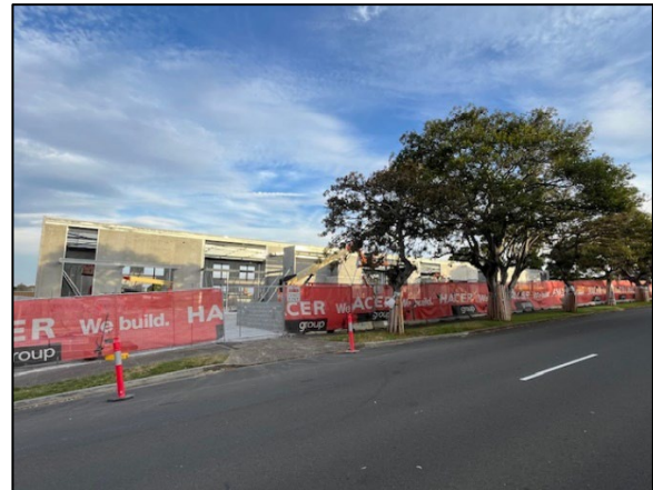
Figure 2: Photo of the subject site (as viewed from Catherine Street)
