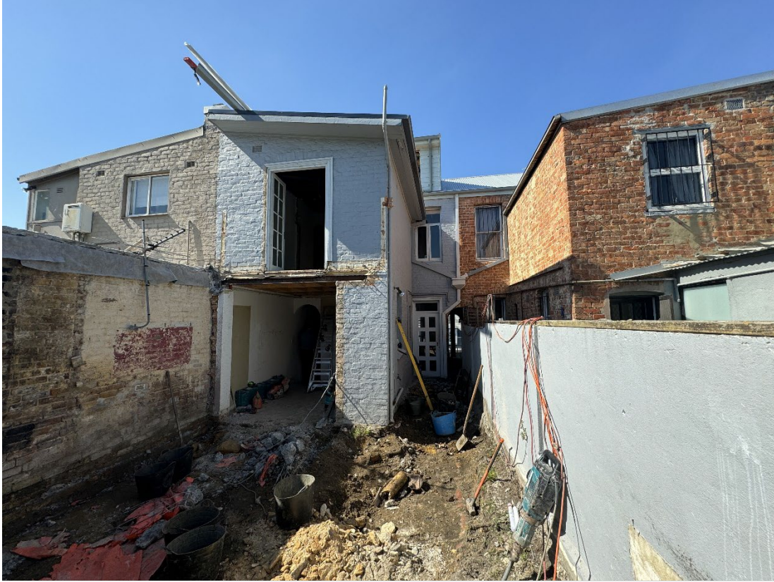
Photo 1: Photo taken from rear of property looking south
