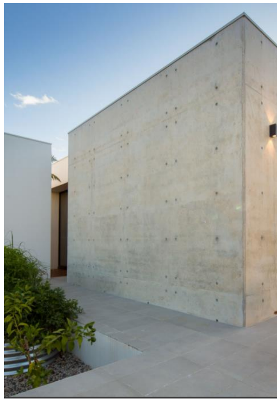
FM1- OFF FORM CONCRETE
