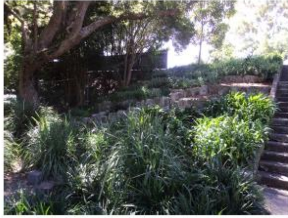
Figure 3-19 Interwar stone edging, retaining walls and stair at the northwestern corner of the Park.
