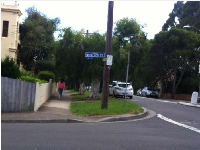
Figure 4-9: Hawthorne Pde / Tressider Ave Intersection – Missing Pram Ramp
