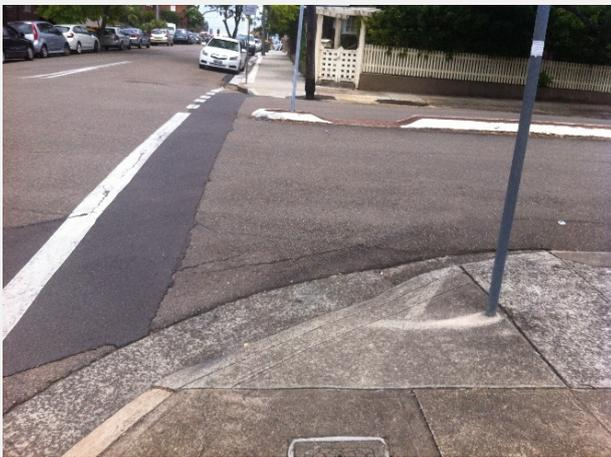
Figure 4-8: Holden St / Palace St Intersection (North-west Corner) – Non-Standard Ramp
