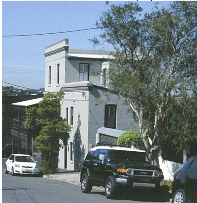
Photo 3: View of existing building from Smith Street.
