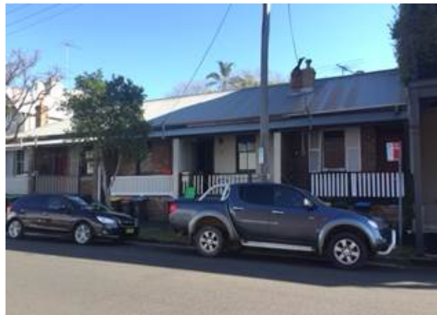
Photo 2: View of adjoining dwellings as viewed from Mansfield Street.
