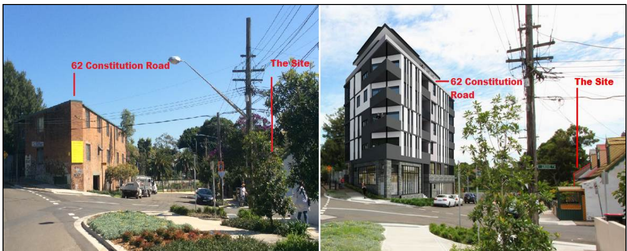
Image 7: Existing warehouse and approved 7 storey development – 62 Constitution Road
