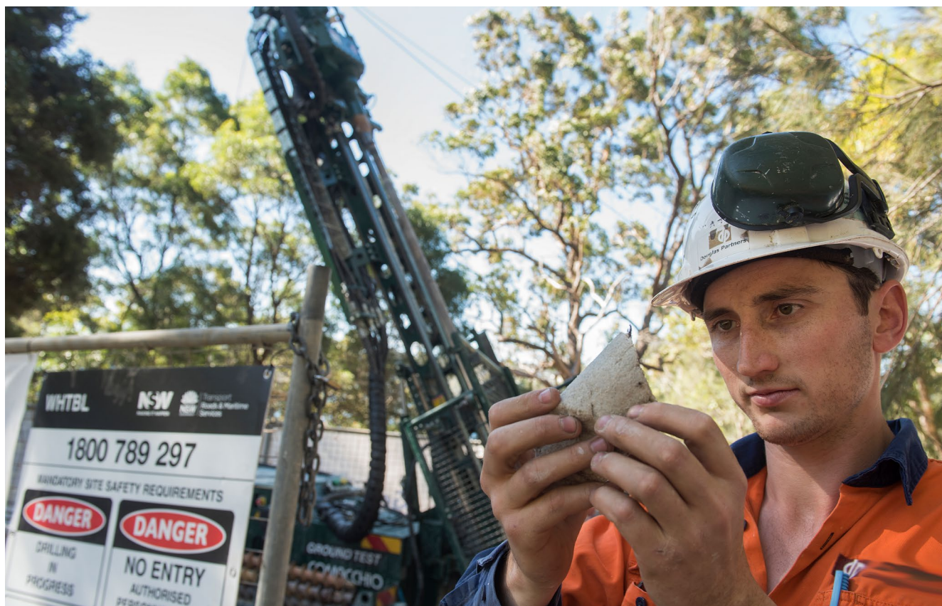
Geotechnical test drilling at Northbridge
