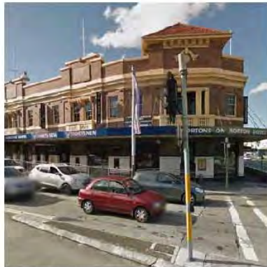
The heritage listed Horton Hotel marks the entry to Norton Street from Paramatta Road
