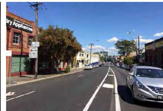
Plymouth Bridge Road forms a main spine to the Precinct, running east-west between Booth Street and Parramatta Road.
