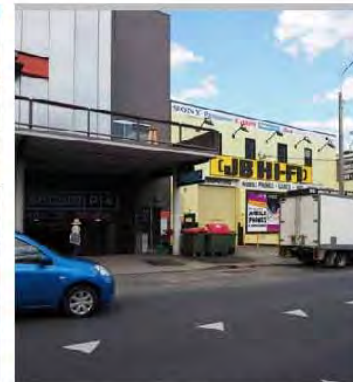
The eastern edge is characterised by large blocks, poor built form and low footpath amenity with many driveway entries
