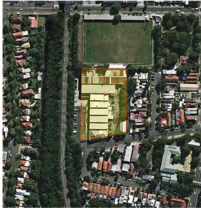
Figure 1: Aerial view of the subject site
