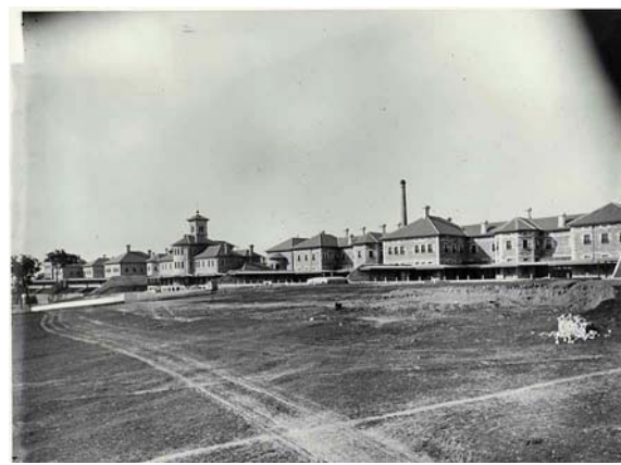
Figure 2-6 Kirkbride Block viewed from the southwest, circa 1883 Source: State Records Series 4481, Image 941
