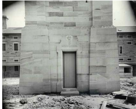
Figure 2-18 Base of Tower, circa 1883 Source: State Records Series 4481 Image 949
