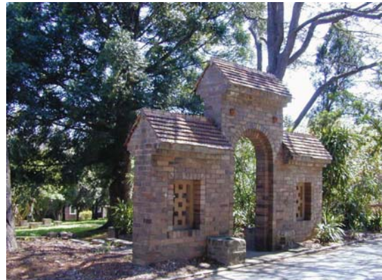
Figure 2-41 Garden edging tiles from the Keep garden were used as roof tiles for the ornamental gateway. Source:
