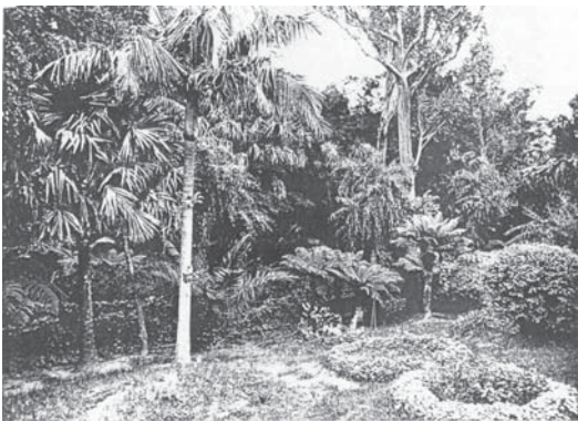
Figure 2-38 Broughton Hall, 1900. Source:
