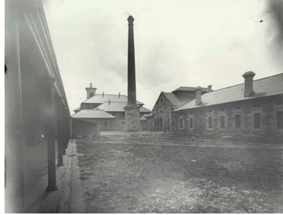
Figure 2-16 Boiler House and flue, circa 1883 Source: State Records Series 4481 Image 950
