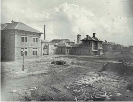
Figure 2-11 Kirkbride Block viewed from the southeast, circa 1883 Source: State Records Series 4481 Image 951
