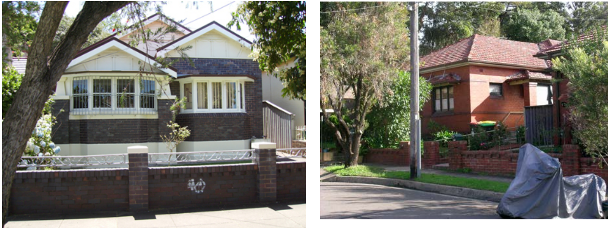
Figure 1: Examples of Inter-War period housing styles in Marrickville HCAs. Note use of matching brickwork for front fences. Both of these examples have side entries.
