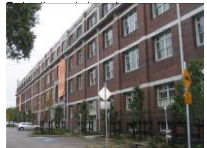
Federation period warehouse
