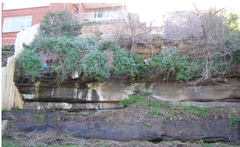
Managing development close to rock overhangs is important for environmental and scenic quality reasons and safety and geotechnical considerations. Water run off from properties will, overtime, destabilise these areas if not properly managed.
