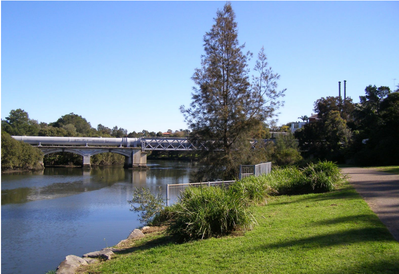
The Cooks River Aqueduct is a State listed heritage item owned by Sydney Water
