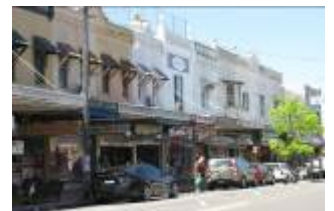
Victorian character of Dulwich Hill shopping centre with interesting silhouette of parapets and awnings unifying the townscape.
