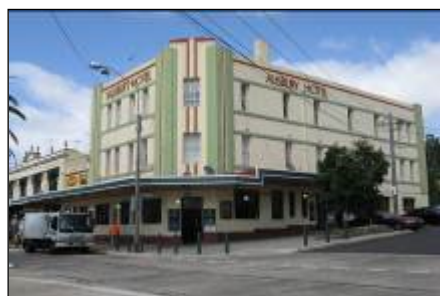
Three storey hotel acts as a marker of the Stanmore commercial centre.
