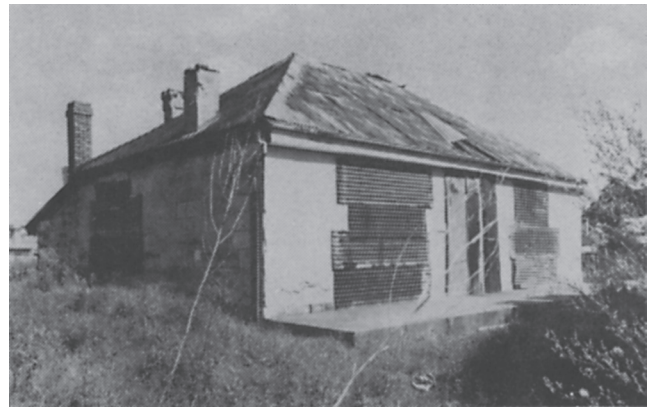
Clontarf, 4 Wallace Street, Balmain now derelict, its verandah destroyed
