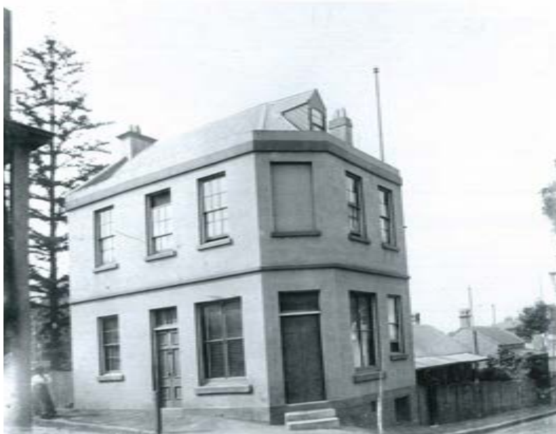
The Old Post Office, 1 Queens Place, c.1850 Nos 2–6 Waterview Street are to be seen. (Balmain Association)
