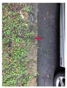
Figure 10 | Concrete patching in the kerb where the veranda post once stood.
