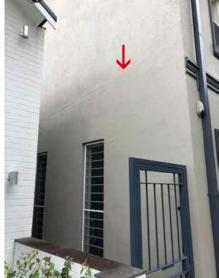
Figure 8 Traces of ashlar scribing on the side. Figure 9 Outline of a removed side skillion in The front elevation was rendered recently with smooth render.
