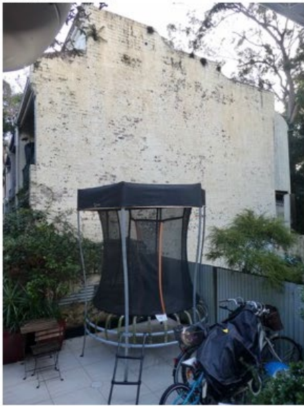
The backyard, with side of terrace at 27 Rose Street beyond
