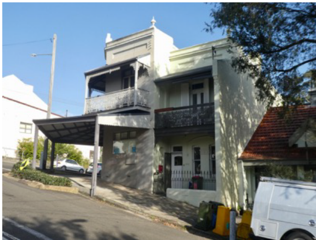
The semi detached terrace style pair, from the north-east
