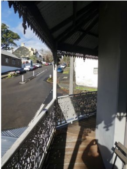
View to south up Trafalgar Street from eastern veranda
