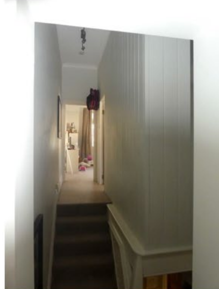
Upper flight of original dog leg stair. Office is behind vertical boarded timber partition.
