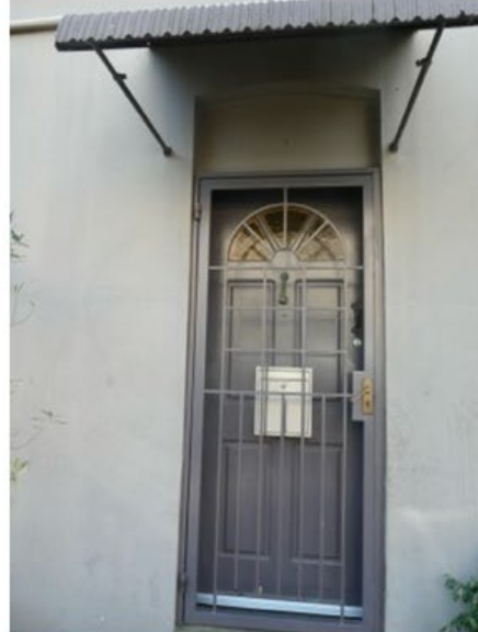
Non-original door on Rose Street with fan light painted over, security grill, and awning installed in 1965
