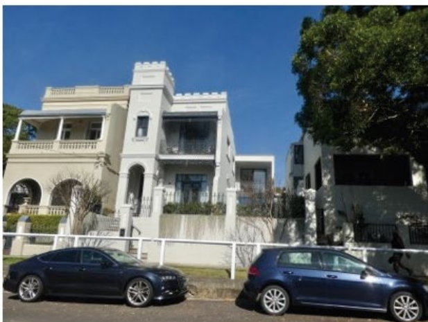
Recent subordinate and complementary contemporary style extension to 20 Rose Street
