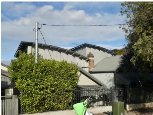
Rear extensions to single storey cottages, View Street
