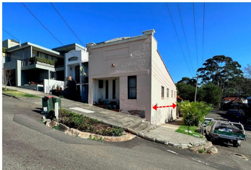
Figure 2: No. 268A Trafalgar Street (to the south)
