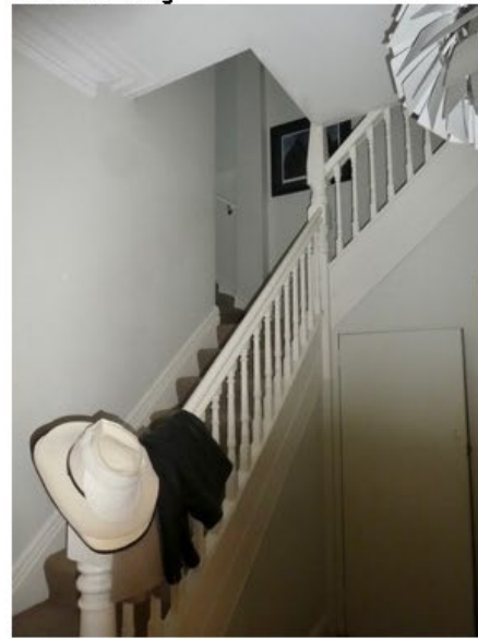
The original staircase
