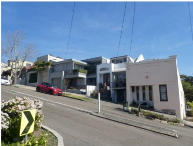
Western side of Trafalgar Street. From right: modified shop on corner of Rose Street; unrecognisably modified Victorian terrace, two late 20th century houses
