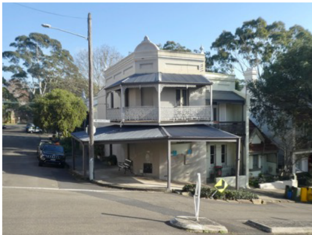
The subject building, from the east
