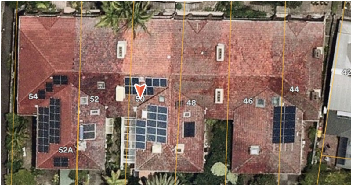
Image 2: Aerial image of No.44 – 54 Glassop Street and matching terracotta roof cladding. Note the solar panels and hot water systems installed on the rear roof planes of Nos. 54, 52, 50, 48 and 44.
