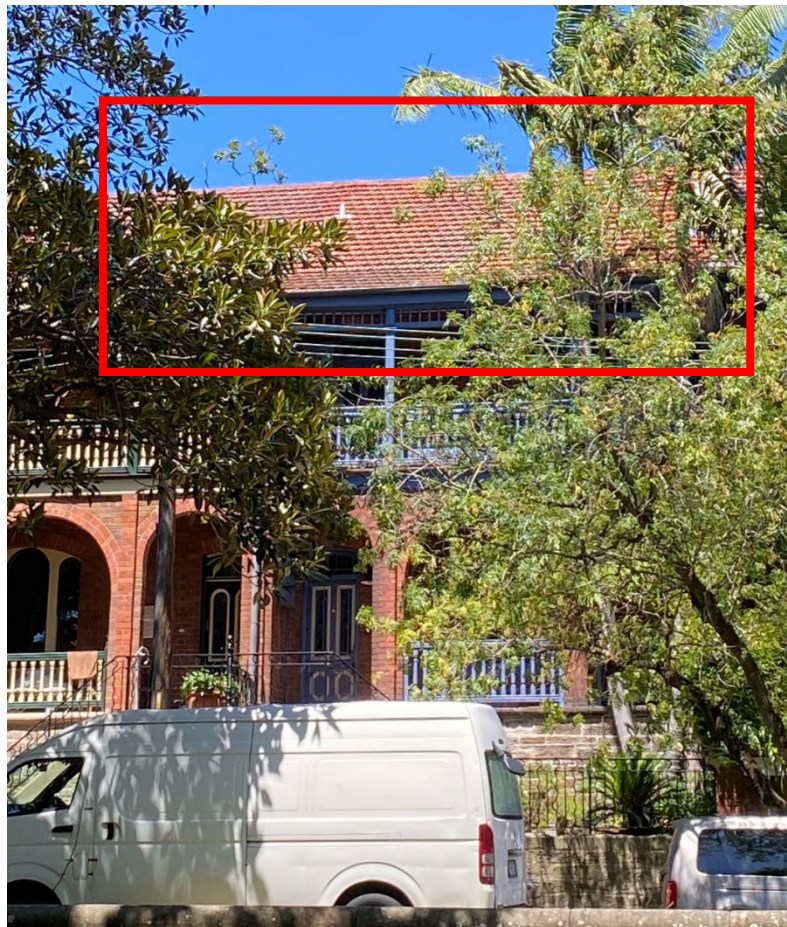
Image 7: Zoomed in view from public park, roof plane subject to the proposal in red.
