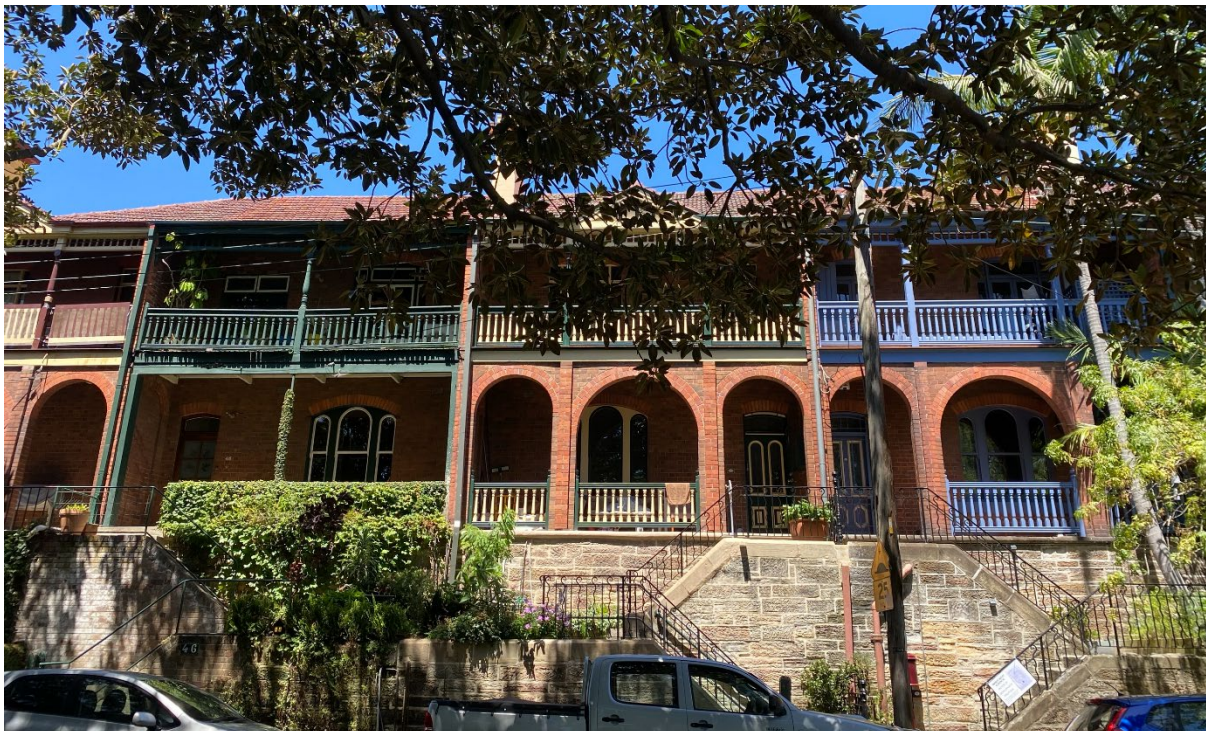
Image 7: front elevation of No. 44 (left) to 50 (right) Glassop Street.
