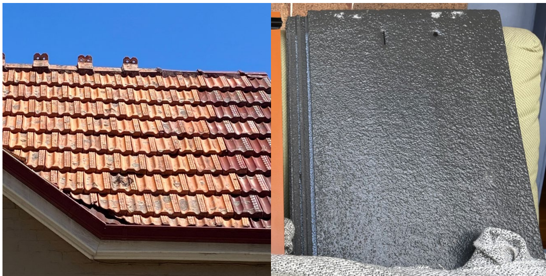
Image 1: Marseille Terracotta Roof Tiles as seen on No. 56 Glassop Street (left), proposed roof tile to be colour-matched terracotta (right)
