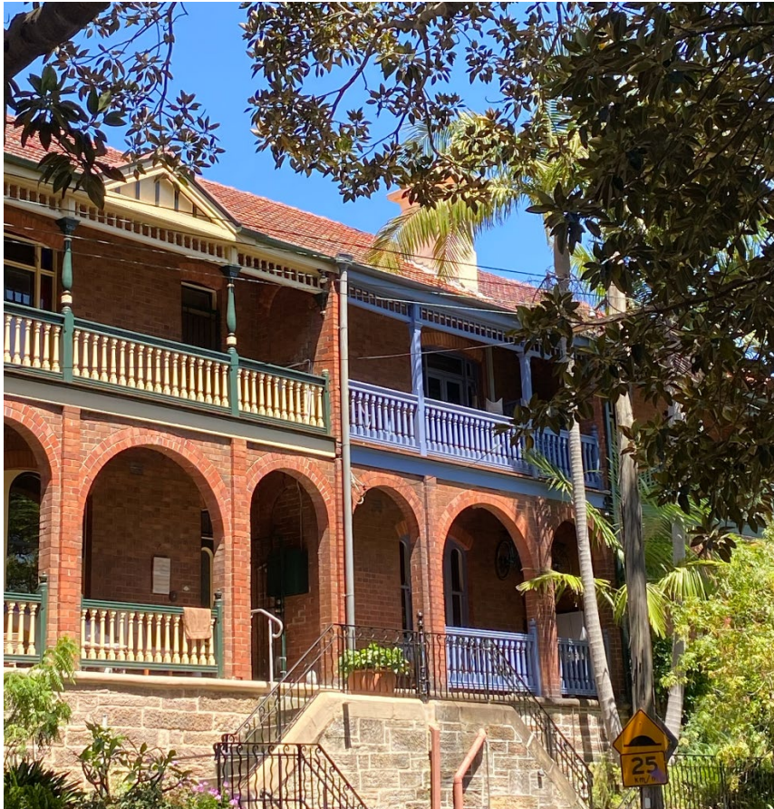
Image 4: subject property (blue railing) from streetscape (north vantage point)
