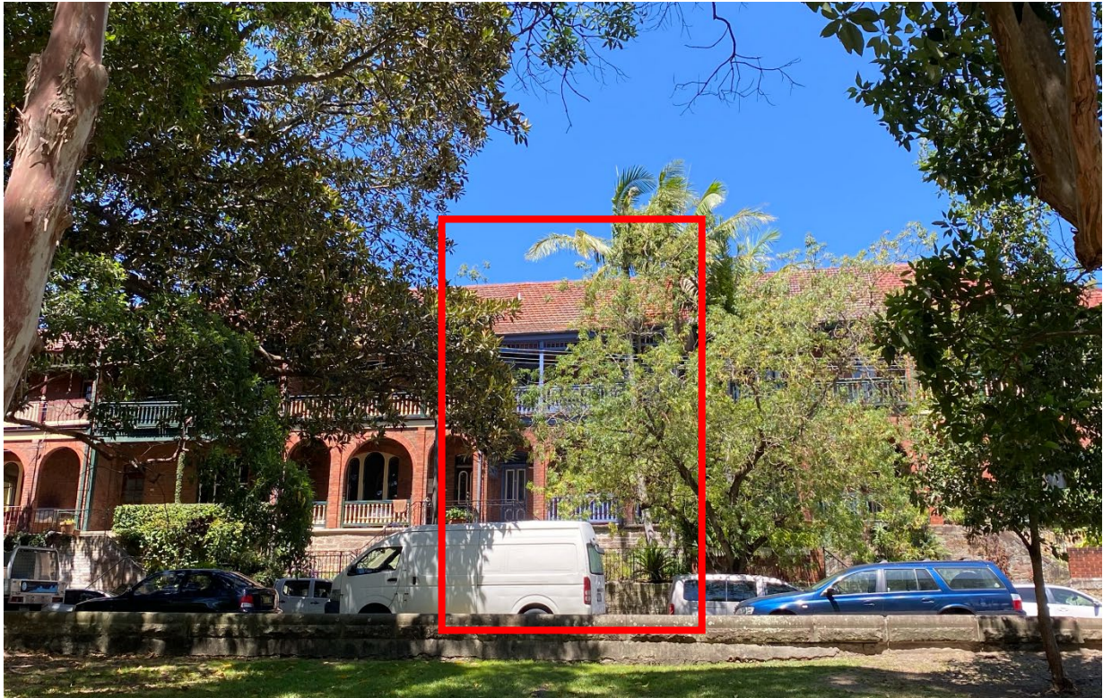
Image 6: View from the public park (Elkington Park), subject site in red box.
