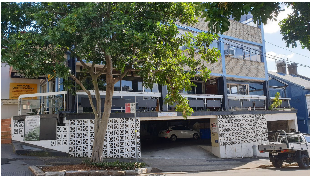
View of existing car parking entry from Church Street
