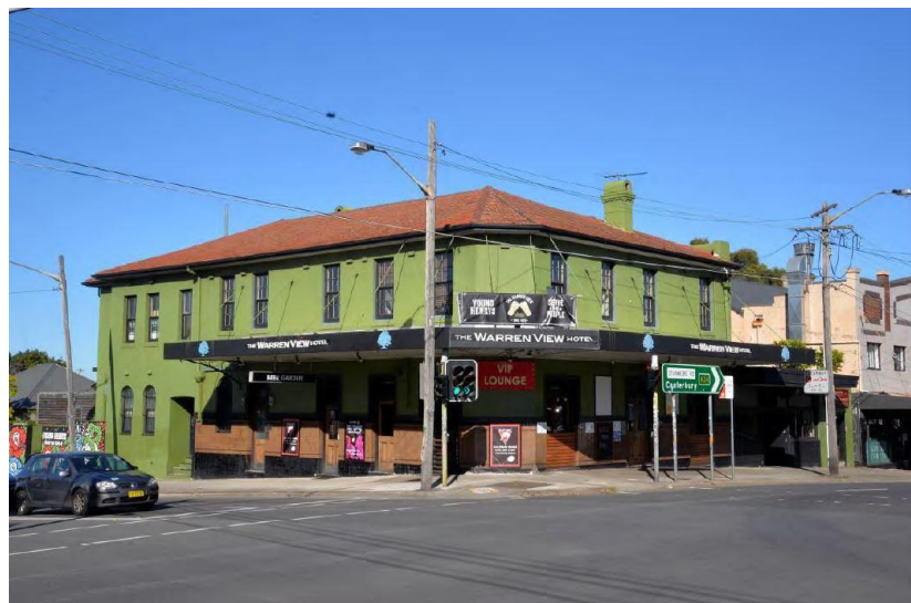
Site 13 – The Milestone Hotel
