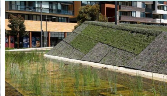
The Drying Green at Green Square, Sydney, has incorporated WSUD in the form of local wetland. WSUD can also be implemented through rain gardens, sediment ponds, swales and rainwater tanks.
