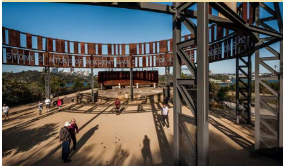
Walama/Ballast Point Park has incorporated design that acknowledges historic remains from when the area was one of Sydney's major oil distribution sites.
