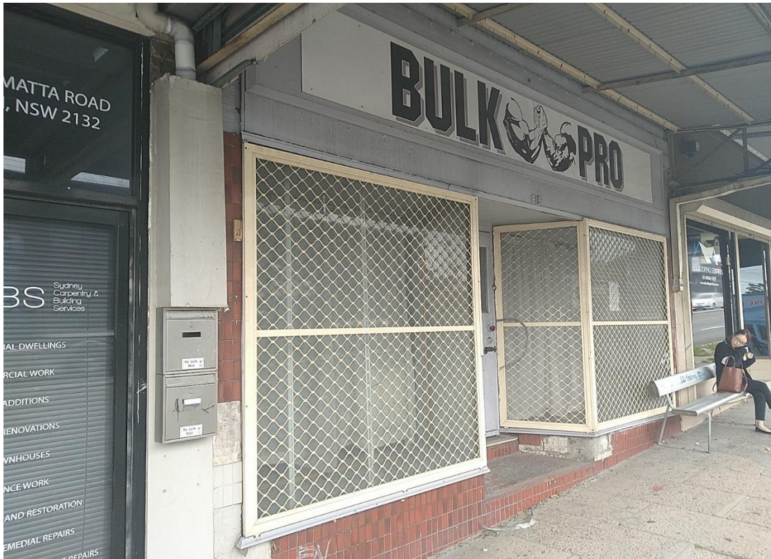
Photograph 1: 616 Parramatta road shopfront (currently vacant)
