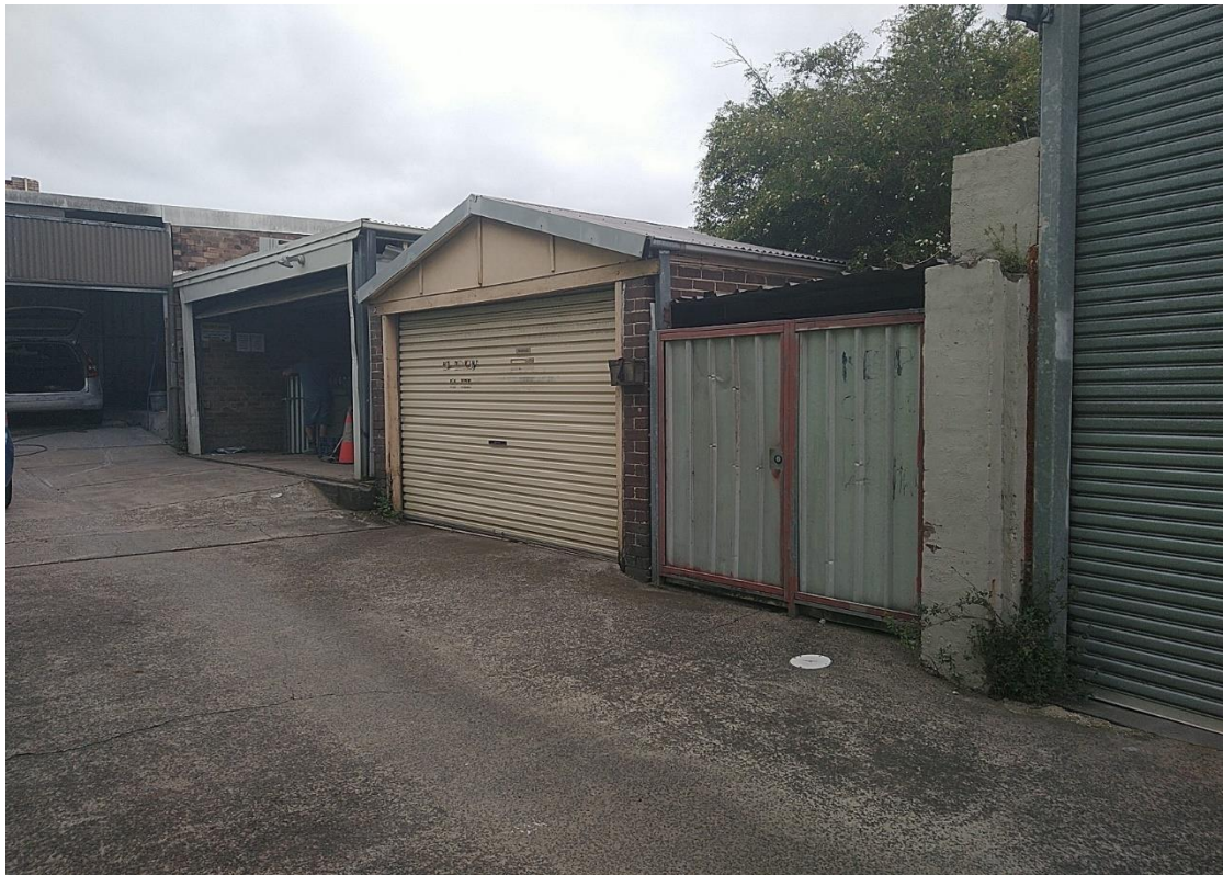
Photograph 2: Rear garages of premises 616-618 Parramatta Road
