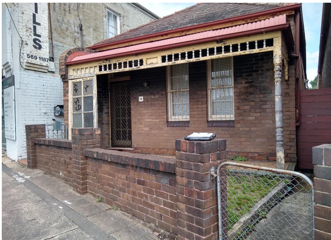
Photo 4: Vacant residential building at 14 Crystal Street
