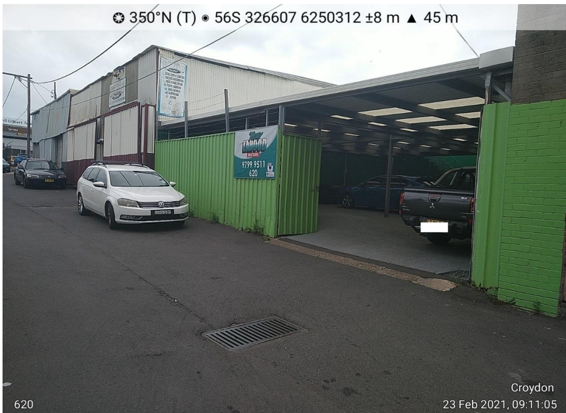
Photo 4: Drainage system at rear of the premises
