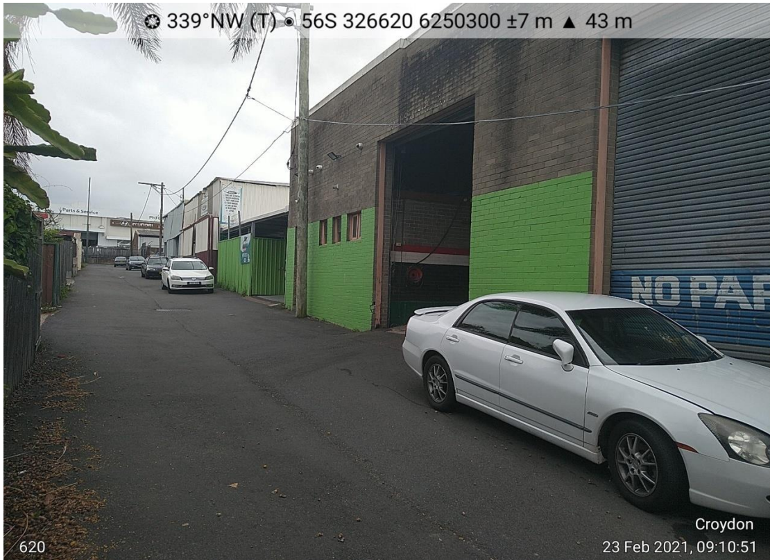
Photo 5: Warehouse building occupying 210 Croydon Road.
