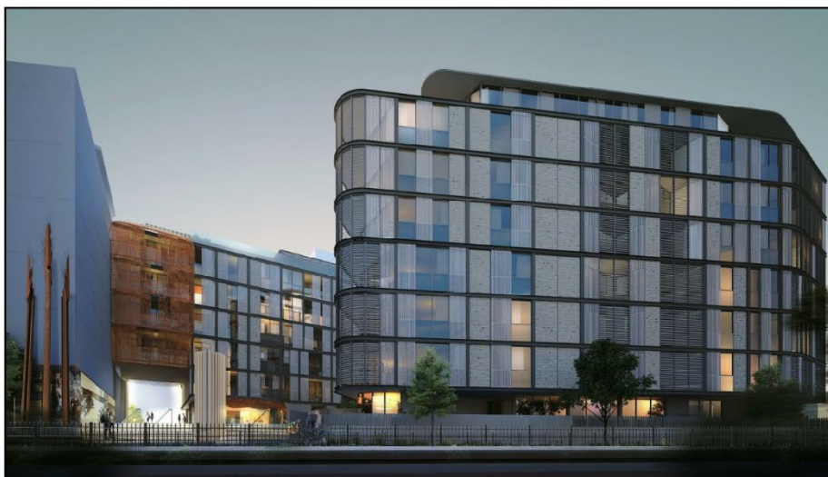
Image 3: No. 4-12 McGill Street as viewed from the greenway corridor to the west of the sites
