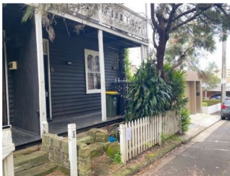
Figure 28: Front garden and ground floor of facade
