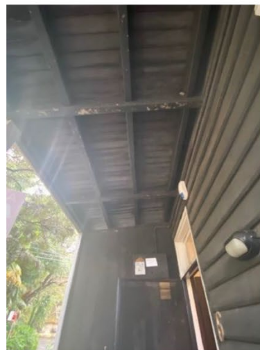
Figure 29: Detailing of weatherboards and verandah
