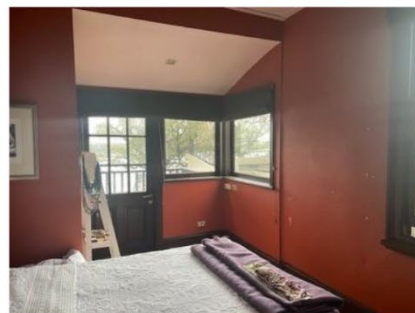
Figure 53: First Floor second bedroom facing south with later addition verandah in view
