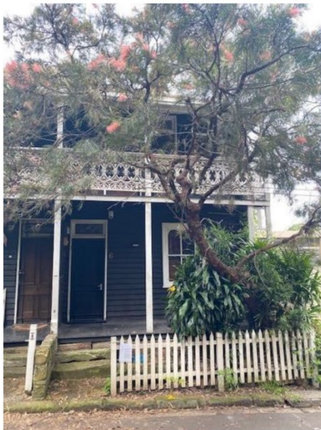
Figure 26: Front façade of No 6 William Street
