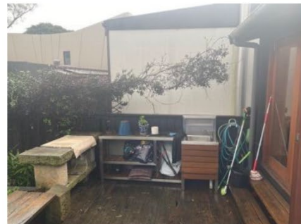
Figure 17: Rear View of 10B from the subject site
