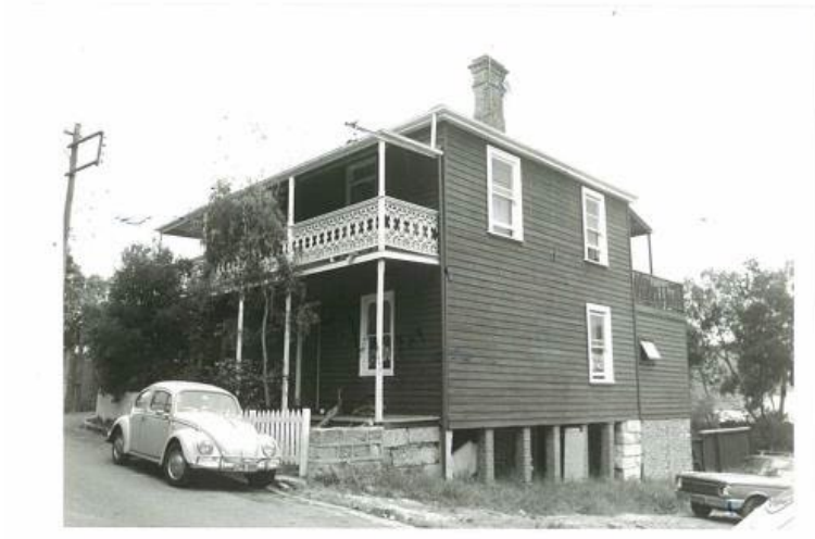
Figure 10: Photo of the building dated 1979 (Source: National Trust)
