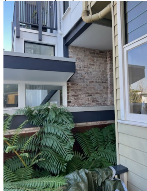
Figure 5 – Rear side elevation of No. 83 Rowntree Street
