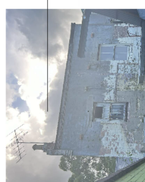
4 Photo south window
