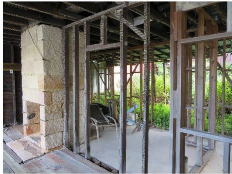
Figure 27 – Looking north-west from corner of dwelling.
