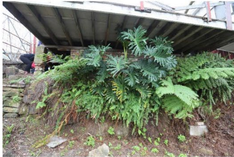
Figure 39 – Overgrown natural rock wall under the contemporary deck.
