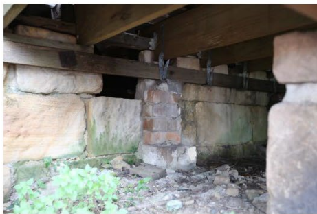
Figure 41 – Sandstone and brick foundations.
