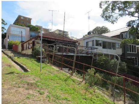
Figure 23 – View north to the subject dwelling from the waterfront end of Johnston Street.
