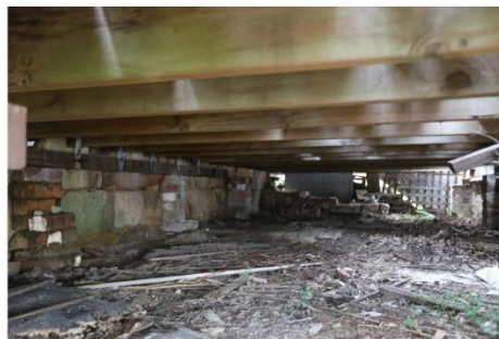
Figure 42 – Subfloor under southern portion of cottage.
