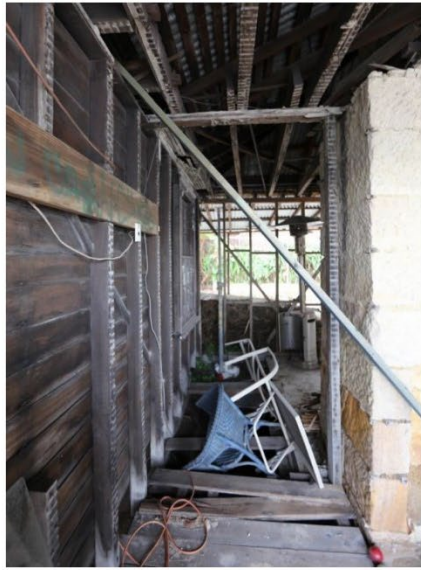
Figure 33 – View north between the fireplace and the western façade.
